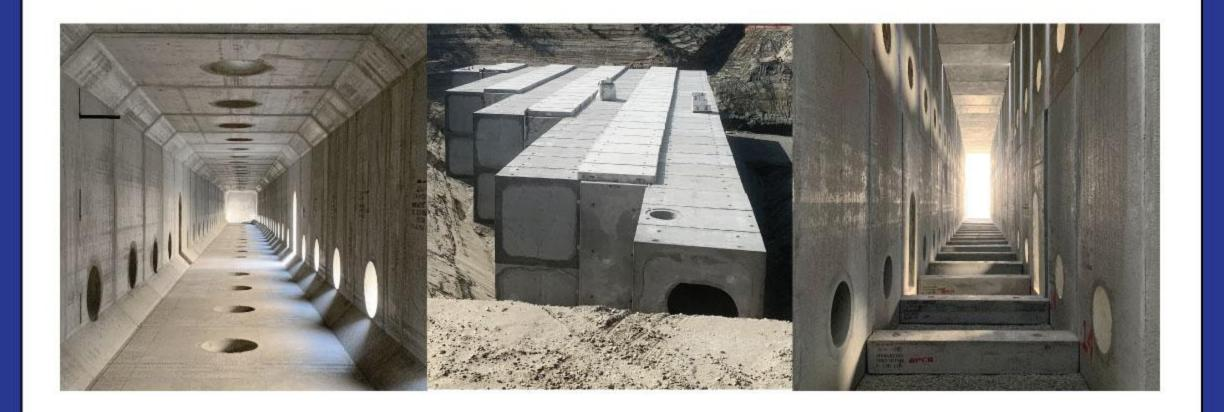
Subsurface infiltration systems are specialized structures installed beneath the ground to capture, treat, and infiltrate stormwater runoff. They act as subterranean reservoirs, collecting and slowly releasing filtered water back into the soil, augmenting groundwater levels, and mitigating surface water pollution. Thus, subsurface infiltration systems are pivotal in enhancing water conservation, improving water quality, and promoting ecological resilience in urban landscapes.
